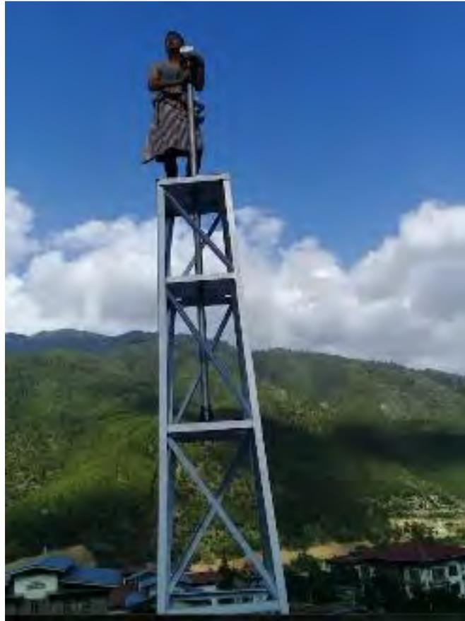
*(Left)* Mr. Dawa of DoTS getting the alignment correct before installing the rotator and stack boom.
