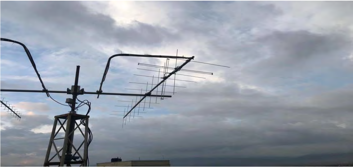
BIRDS VHF Antenna at NAST, used for receiving signal from Satellite NOAA-19
